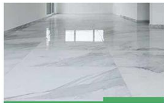
MAINTENANCE MARBLE FLOOR
