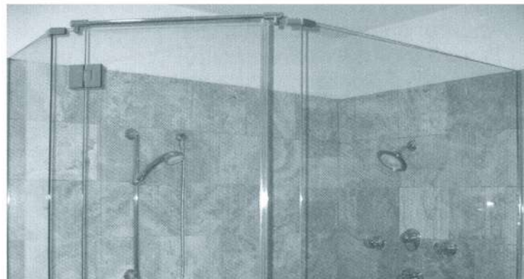
L-2708 Typical Glass-to-Glass Installation Glass-to-Glass Support Bar
